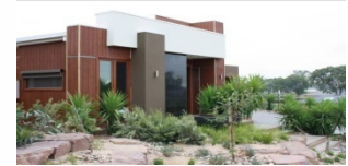
AusZEH Australian First Carbon Neutral Project Home
